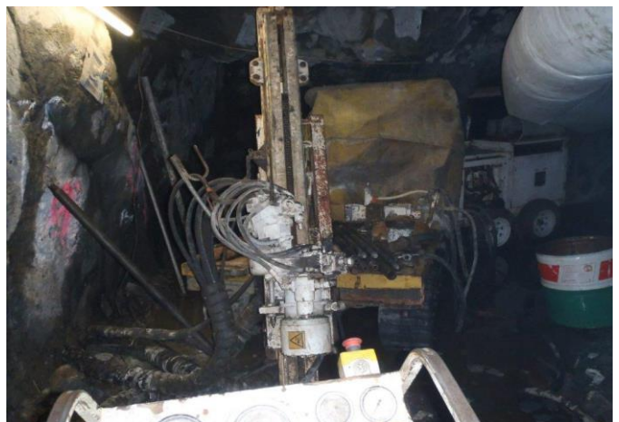
Photo 2 Mobilised drill rig on site at RoD, in adit
