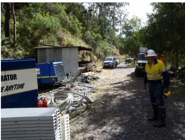
Photo 1 Mobilising Supporting equipment to RoD
