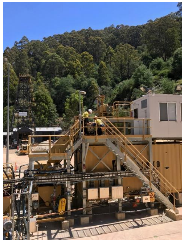
Figure 3. BELOW: Electricians testing process plant circuits prior to testing entire plant.
